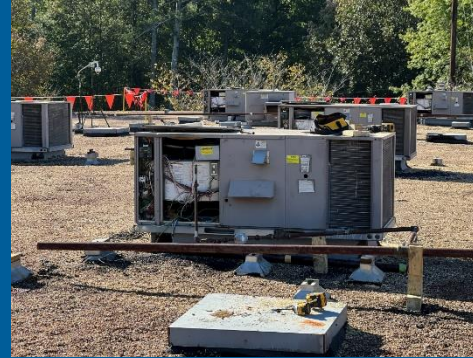
Rooftop Units Disconnected
